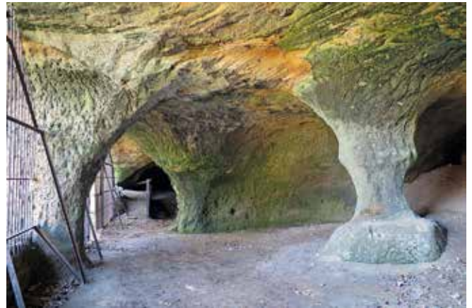
Cemetery Mine: The robbed pillars led to roof falls, resulting in most of the mine being untopped. Photo Clive Penfold
